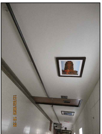
Basement Corridor Looking at Room 14
