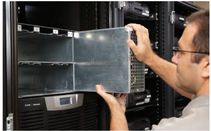
IT staff can easily install electronics modules.
