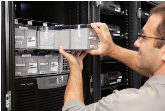
IT staff can easily replace battery modules.
