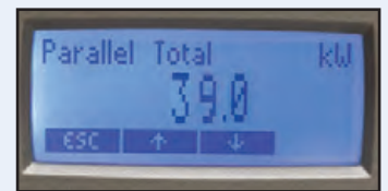
Display full system output from any UPS
