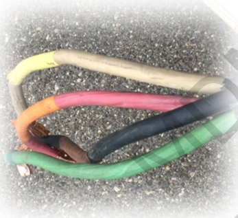
Configuration 4 wire (L1,L2,L3,G) Frequency: 60hz
