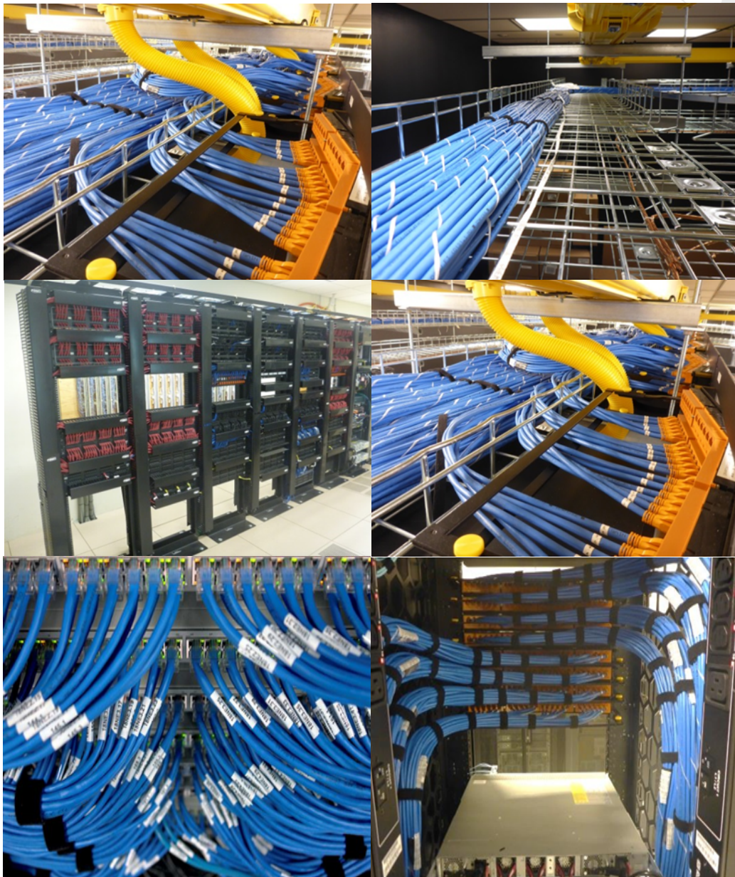
Figure 33: Acceptable Cable Management Results
