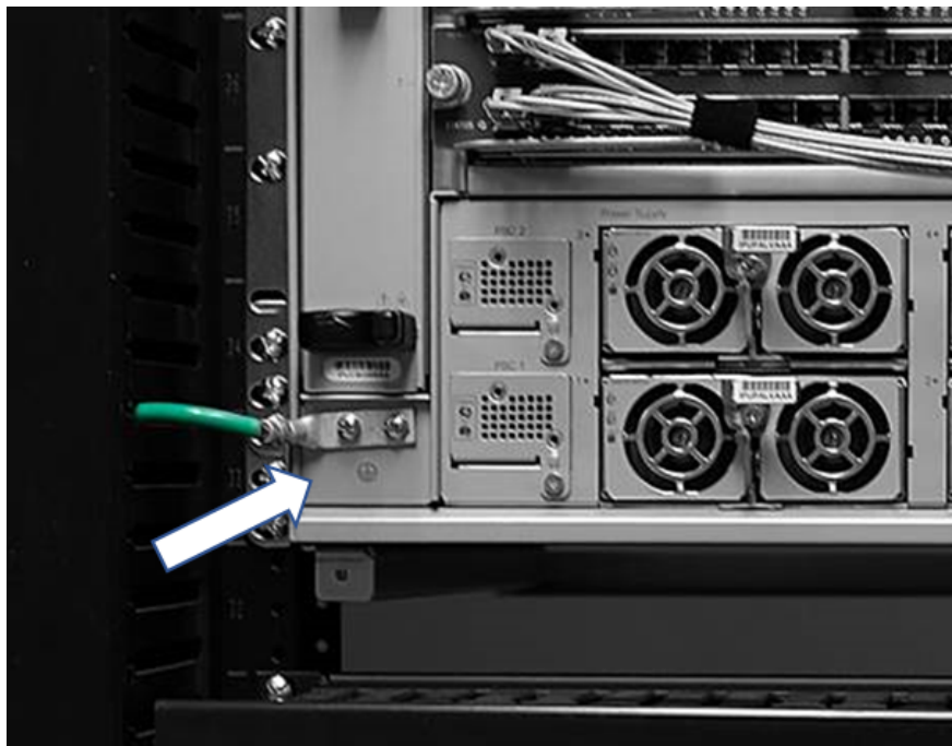
Figure 16: OEM Equipment Ground Connection
