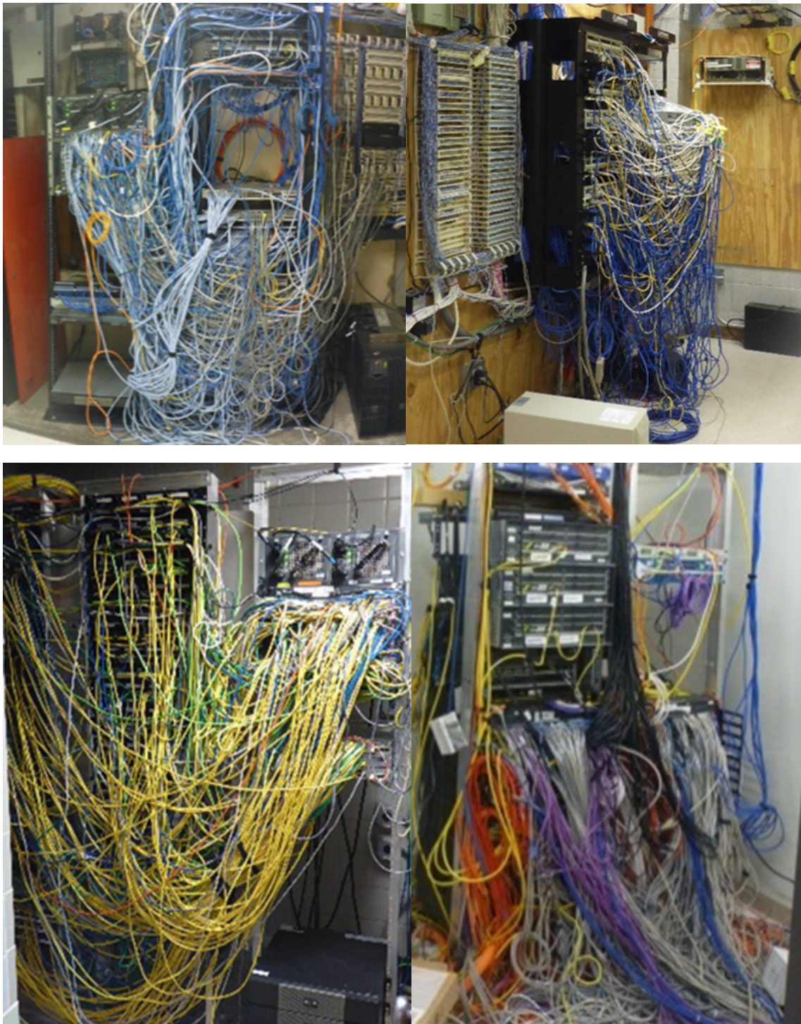
Figure 34: Unacceptable Cable Management Results
