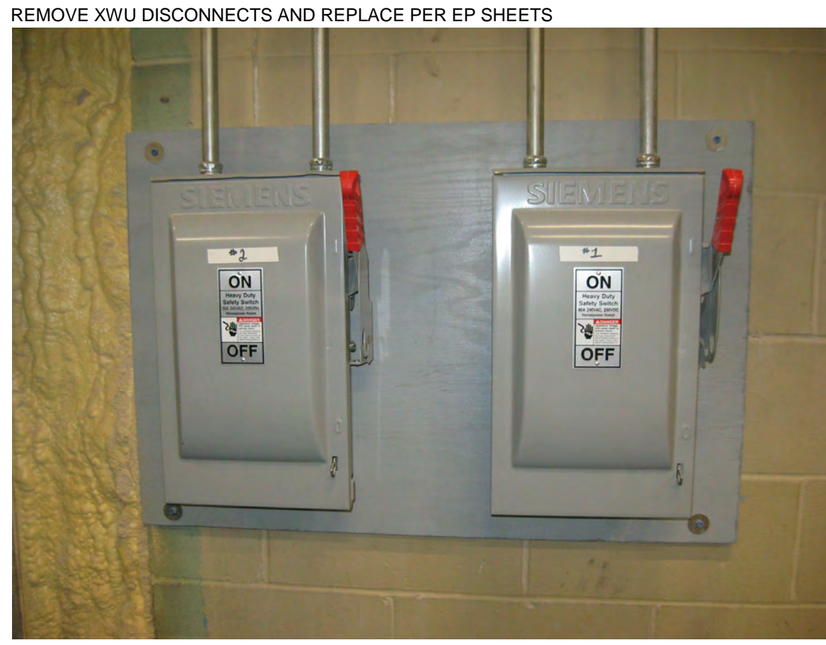
REMOVE XWU DISCONNECTS AND REPLACE PER EP SHEETS 2 WASH EQUIPMENT ROOM: XWU-1,2 DISCONNECTS ED510 N.T.S.
