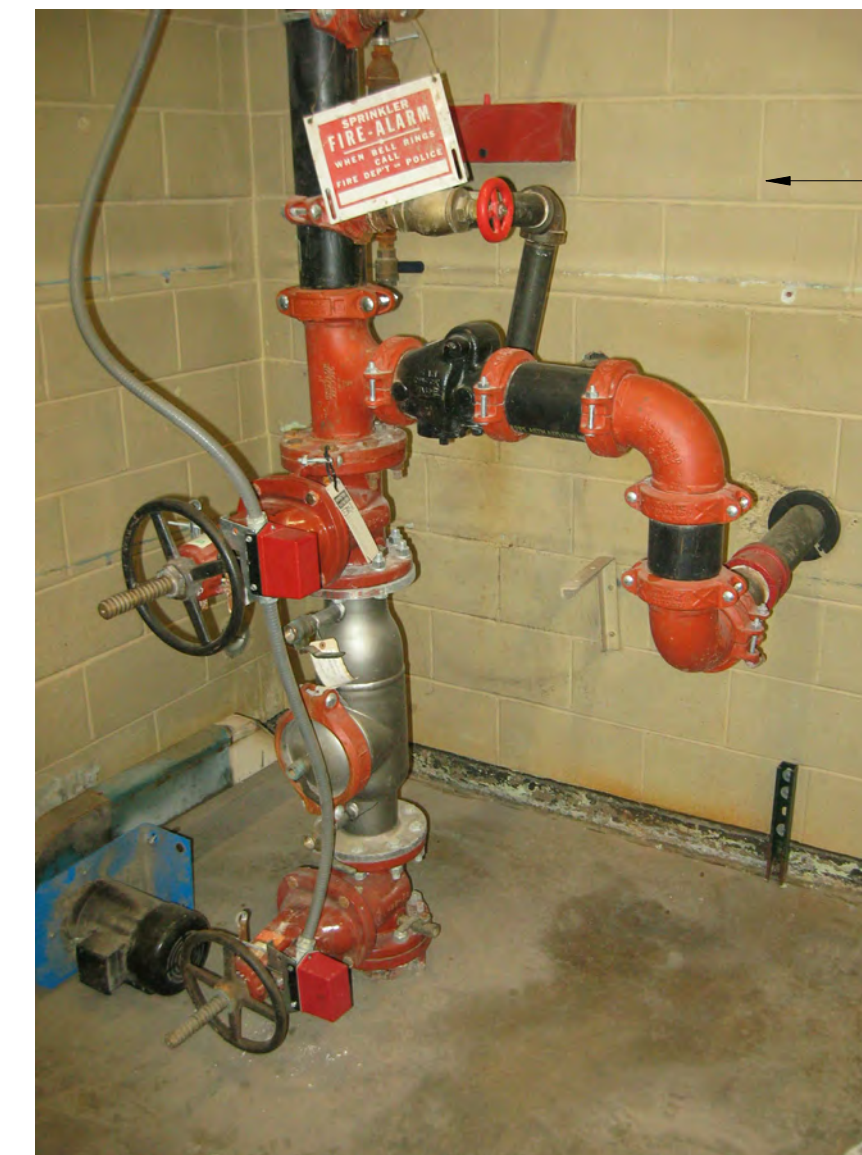
3 WASH EQUIPMENT ROOM: FIRE WATER RISER ED512 N.T.S.
