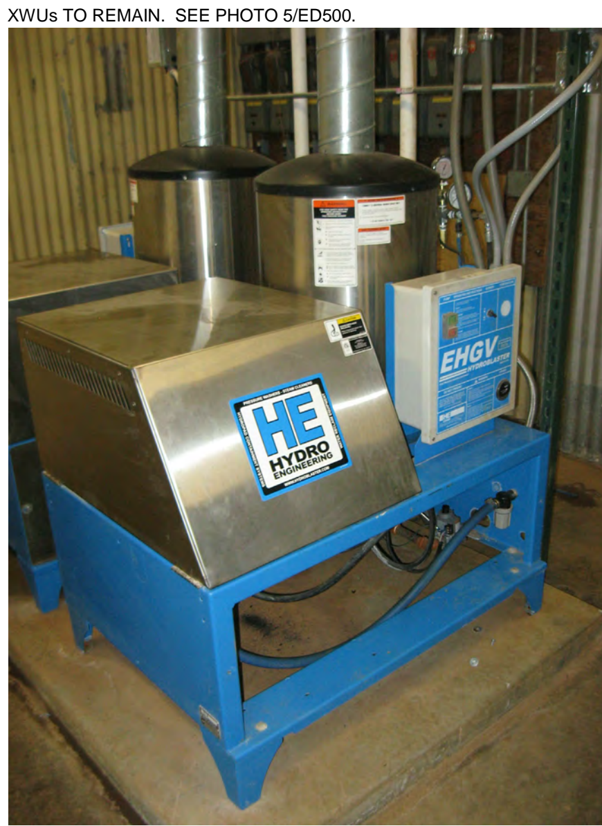
XWUs TO REMAIN. SEE PHOTO 5/ED500. 5 WASH EQUIPMENT ROOM: XWU-3,4 ED510 N.T.S.
