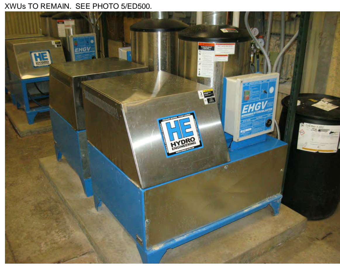
XWUs TO REMAIN. SEE PHOTO 5/ED500. 3 WASH EQUIPMENT ROOM: XWU-1,2 ED510 N.T.S.
