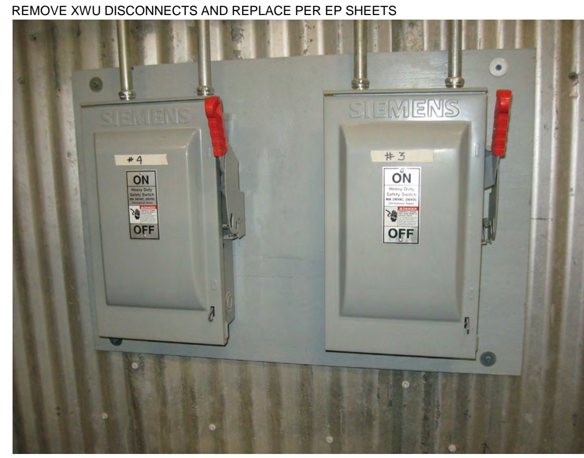
REMOVE XWU DISCONNECTS AND REPLACE PER EP SHEETS 4 WASH EQUIPMENT ROOM: XWU-3,4 DISCONNECTS ED510 N.T.S.
