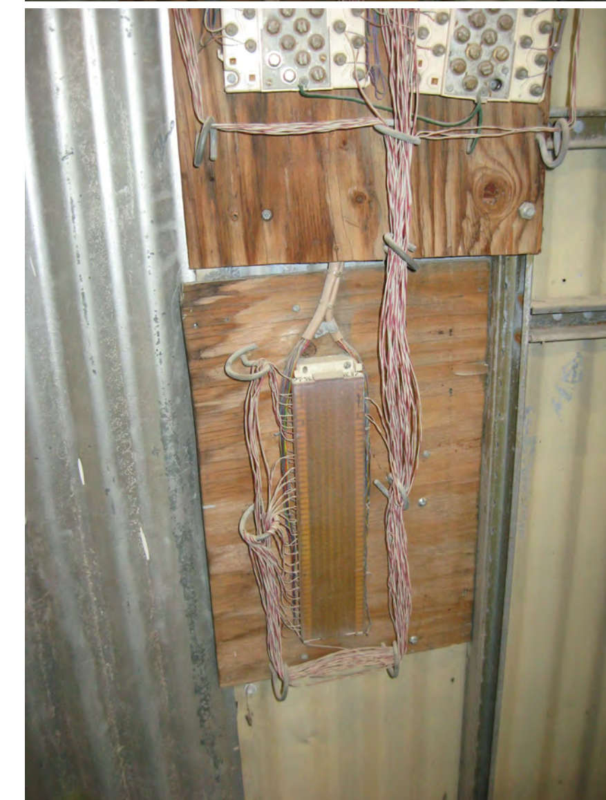
WASH EQUIPMENT ROOM: COPPER COMM ENTRANCE
