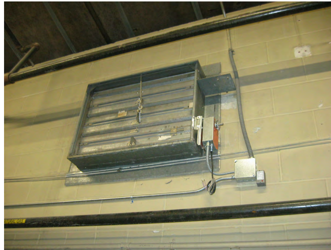
5 WASH EQUIPMENT ROOM: EXHAUST DAMPER ED512 N.T.S.
