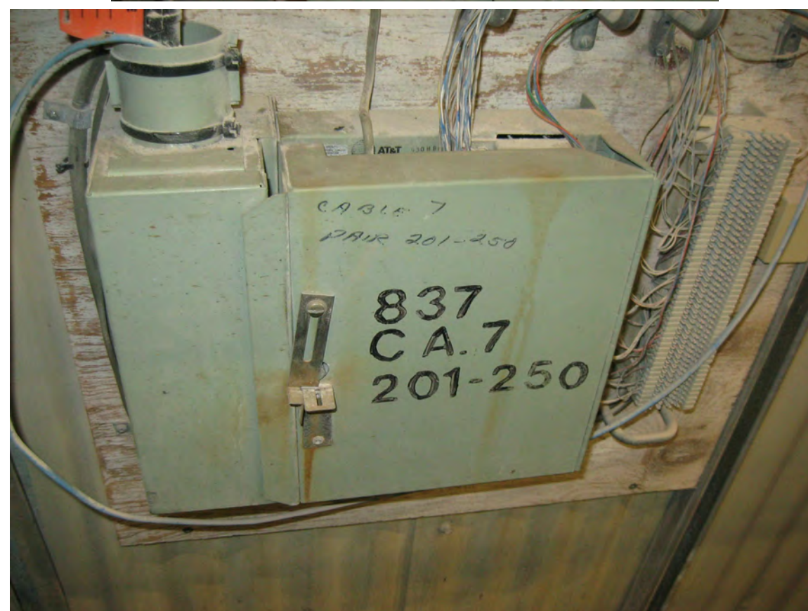
WASH EQUIPMENT ROOM: COPPER COMM ENTRANCE
