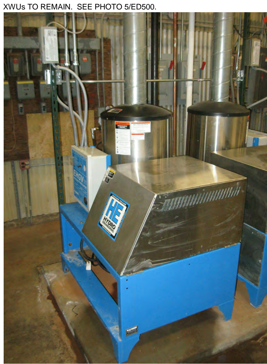
XWUs TO REMAIN. SEE PHOTO 5/ED500. 6 WASH EQUIPMENT ROOM: XWU-3,4 ED510 N.T.S.
