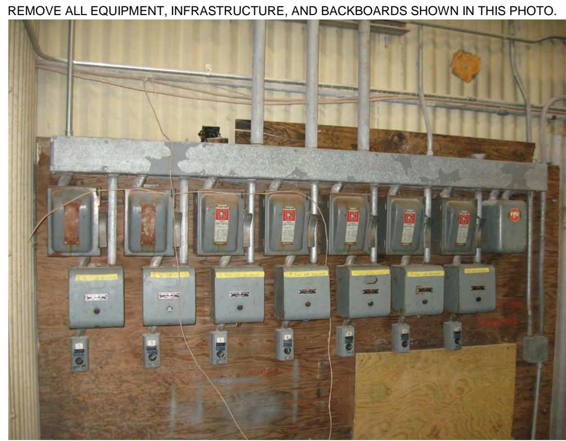
REMOVE ALL EQUIPMENT, INFRASTRUCTURE, AND BACKBOARDS SHOWN IN THIS PHOTO. 7 WASH EQUIPMENT ROOM: HEATER STARTERS ED510 N.T.S.
