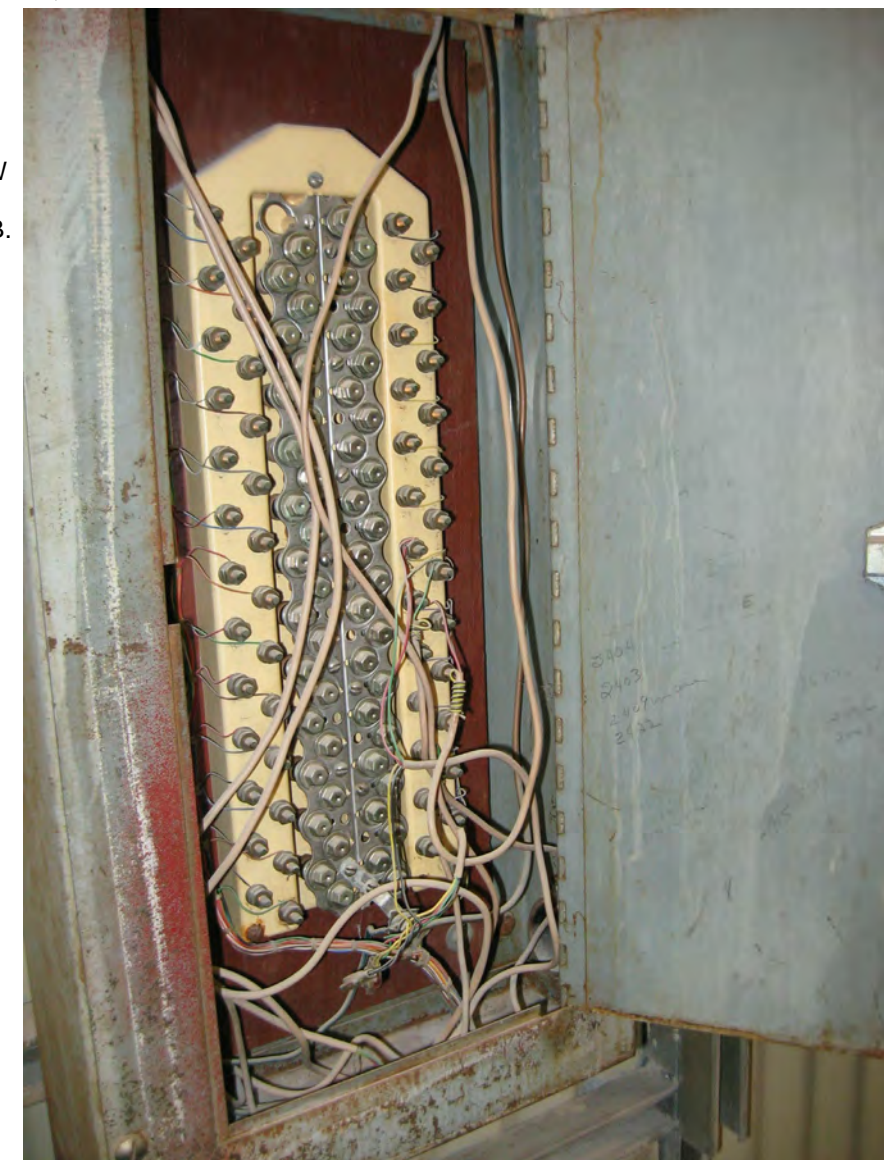
WASH EQUIPMENT ROOM: COPPER COMM ENTRANCE
