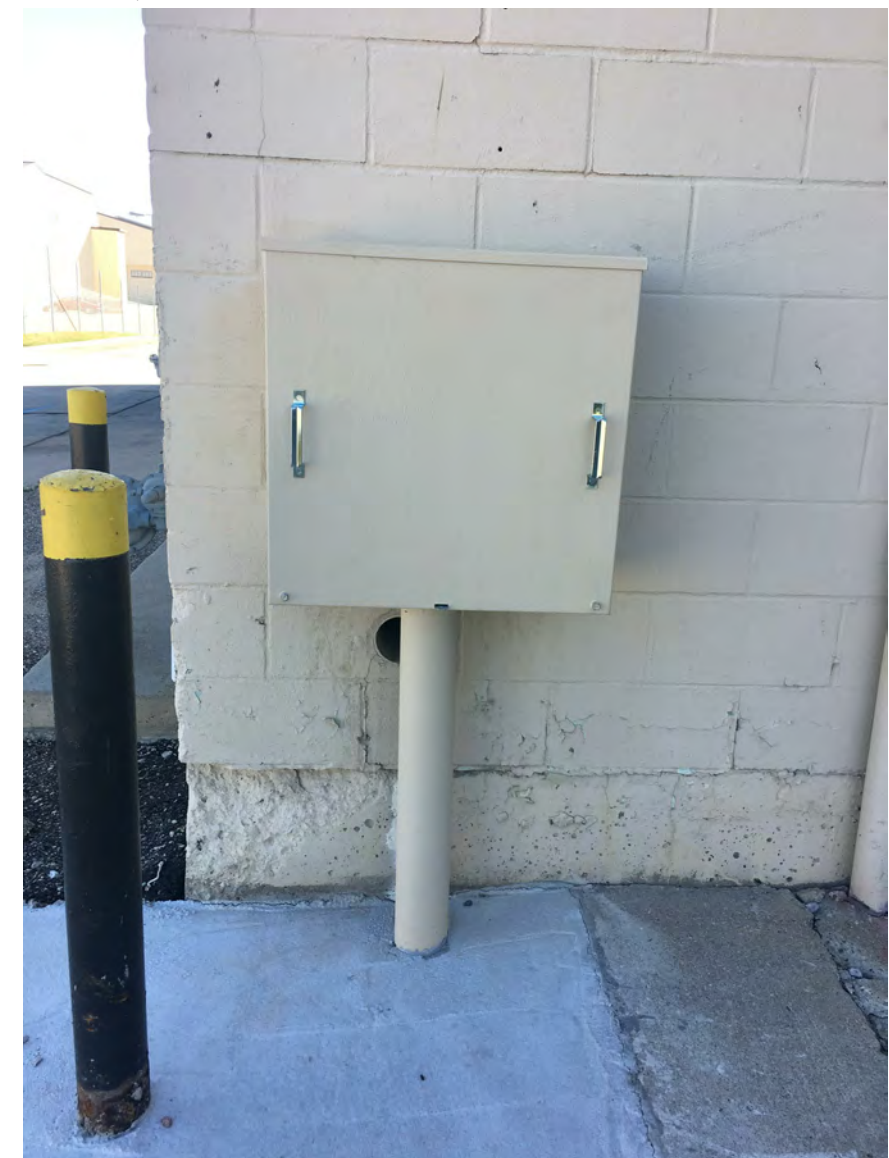
WASH EQUIPMENT ROOM: FIBER COMM ENTRANCE
