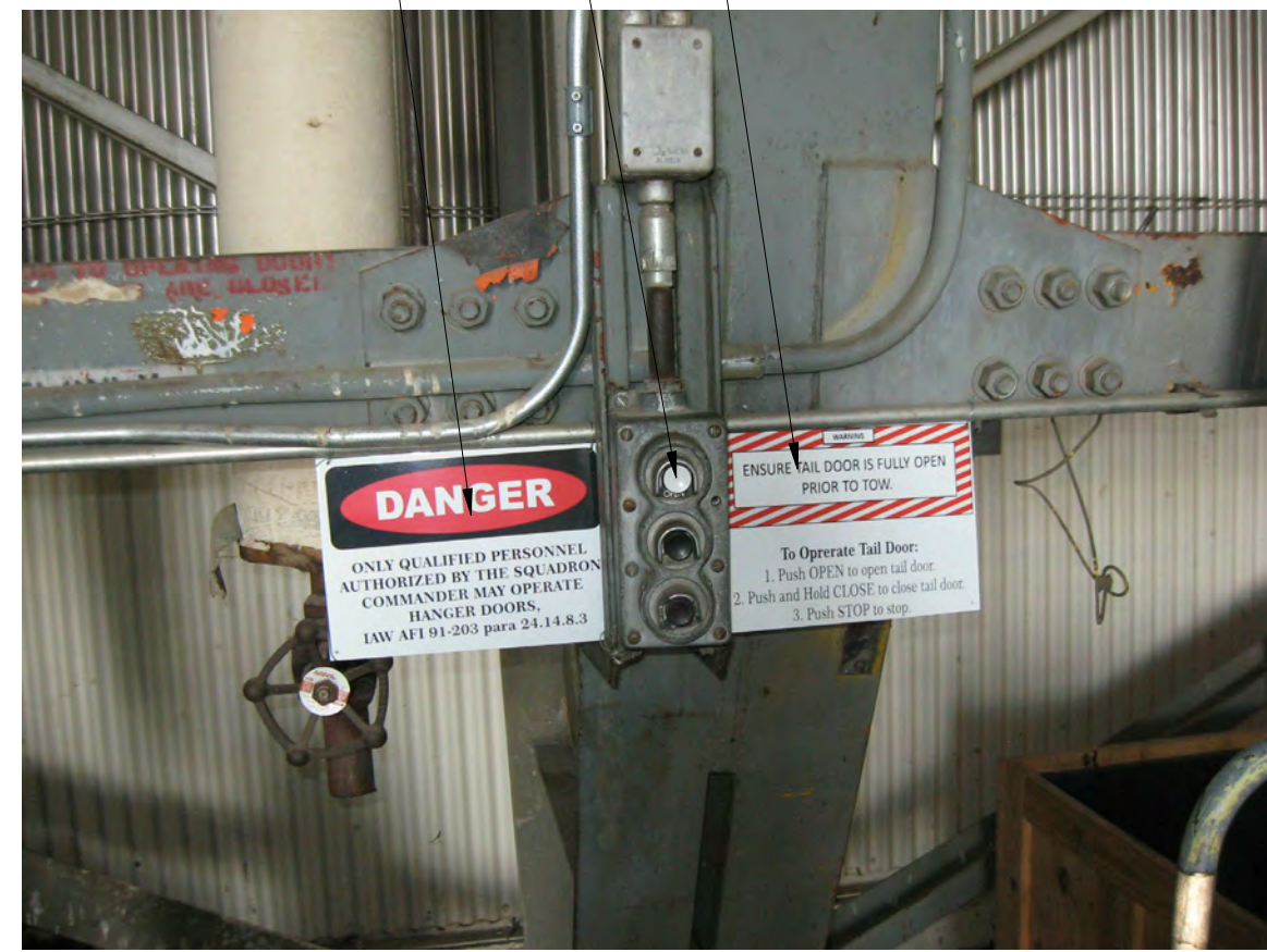
1 HANGAR BAY: TAIL DOOR CTRLS ED500 N.T.S.
