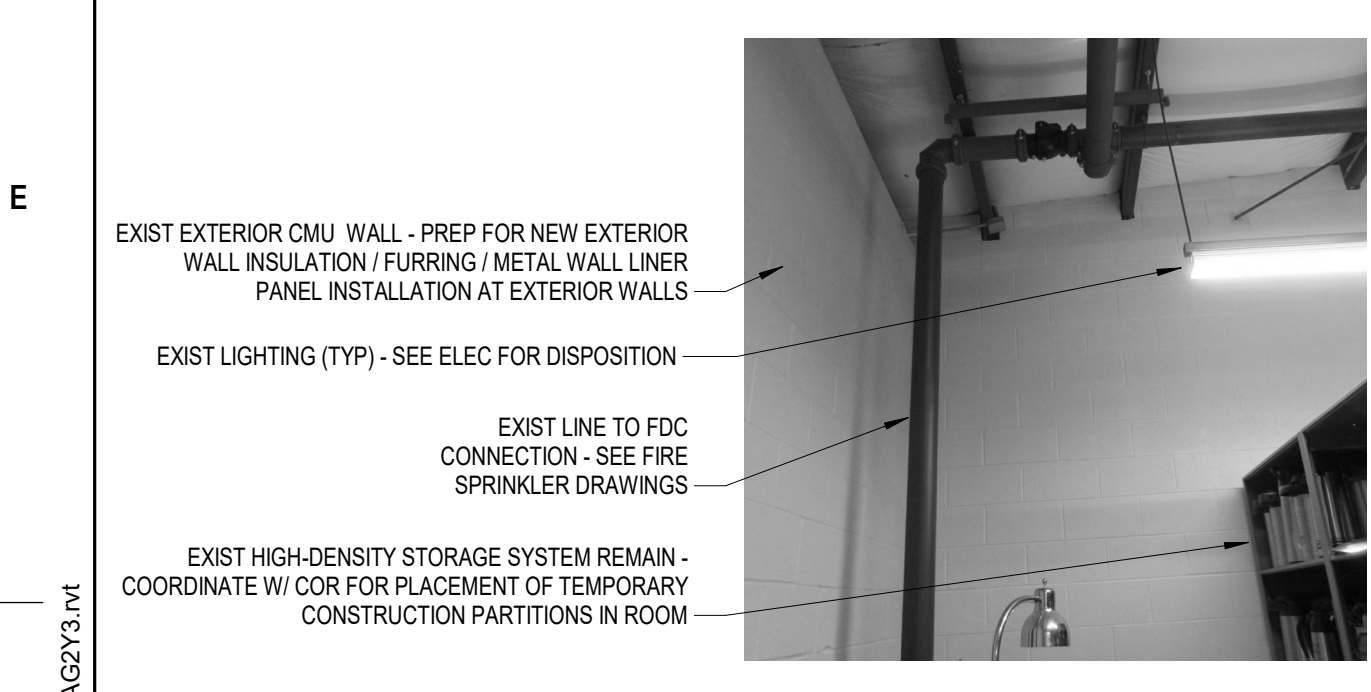
N RM. W01 SW CORNER-FIRE RISER NOT TO SCALE
