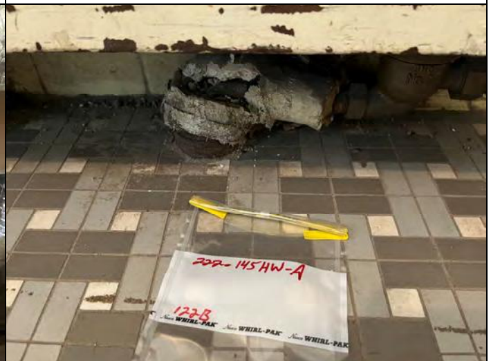
Photo 4 – Samples 222-145HW-A, B, C, asbestos containing 0-4" hard white pipe fittings in building 145 room 122B.
