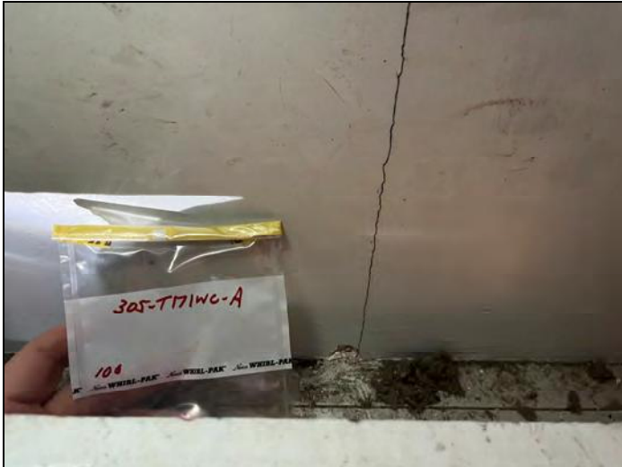
Photo 19 – Sample 305-T171WC-A, less than 1% asbestos containing sheetrock and taping compound walls and ceilings in building T171 room 100.
