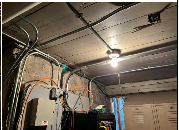
Photo 24 – Test 96, lead containing gray wood ceiling in building 50 room B101.
