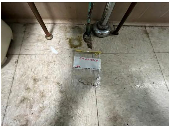
Photo 5 – Sample 310-145TGS-A, asbestos containing (ACM) 12" tan with gray streaks floor tile in building 145, room 132. Only mastic contains.
