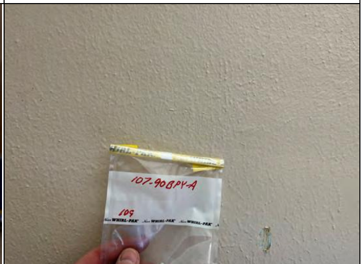
Photo 18 – Samples 107-90BPY-A, B, C, less than 1% asbestos containing bumpy textured walls in building 90 room 109.
