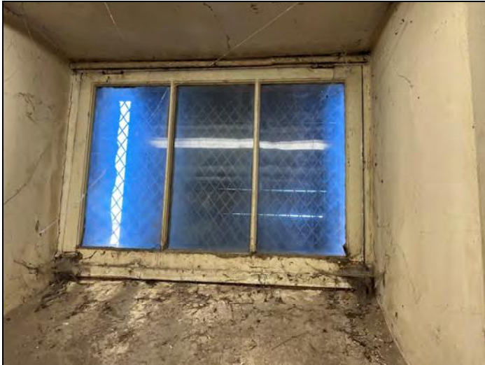
Photo 25 – Test 105, lead containing white window/frame in building 53 room B108.
