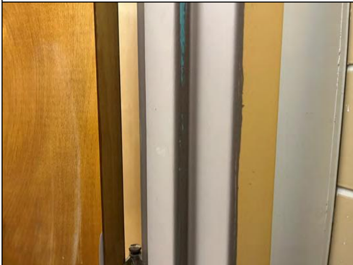
Photo 21 – Test 25, lead containing tan terra cotta block walls in building 145 room TC3A.
