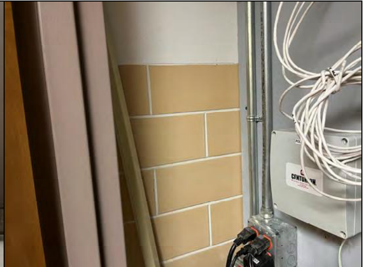
Photo 20 – Test 18, lead containing tan terra cotta block walls in building 145 room TC2A.
