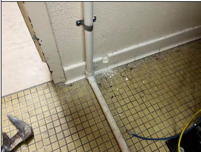
Photo 27 – Test 133, lead containing 6" white ceramic base cove in building 148 room ATC2.
