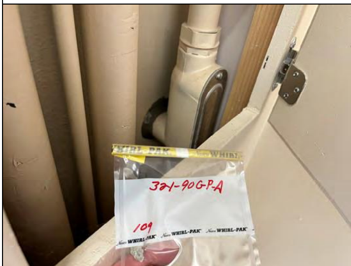
Photo 15 – Sample 321-90GP-A, asbestos containing gray penetration caulking in building 90, room 109.
