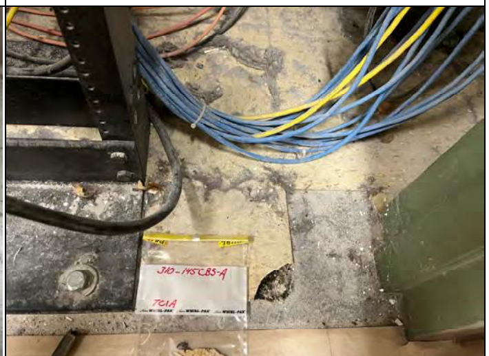
Photo 6 – Sample 310-145CBS-A, asbestos containing 12" cream with brown streaks floor tile in building 145, rooms TC1A and 137C. Only mastic contains.
