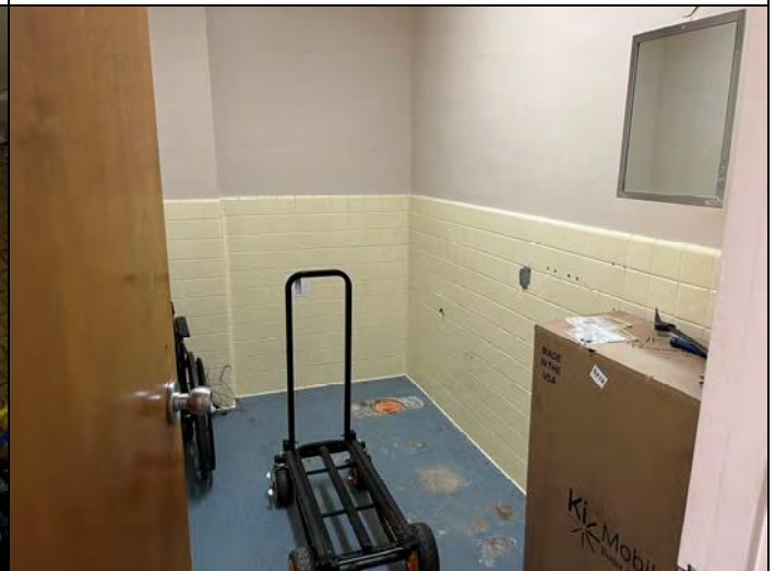
Photo 28 – Test 221, lead containing 4" light yellow ceramic wall tile in building 113 room 169A.
