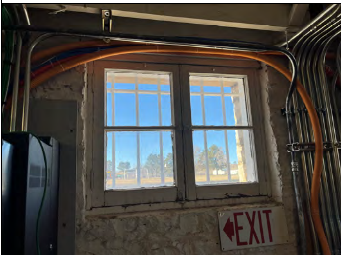
Photo 23 – Test 80, lead containing white wood window in building 46 room B101.
