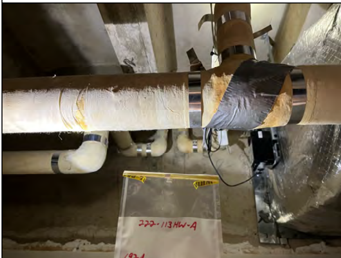
Photo 3 – Samples 222-113HW-A, B, C, asbestos containing 0-4" hard white pipe fittings in building 113 room 192A.
