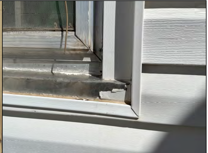
Photo 26 – Test 117, lead containing white metal window frame on building T296 room exterior.
