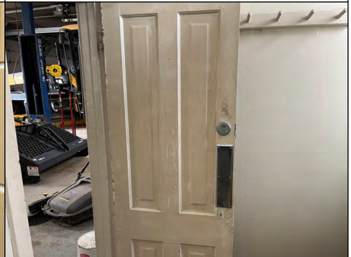
Photo 22 – Test 75, lead containing tan wood door and frame in building T171 room 101B.
