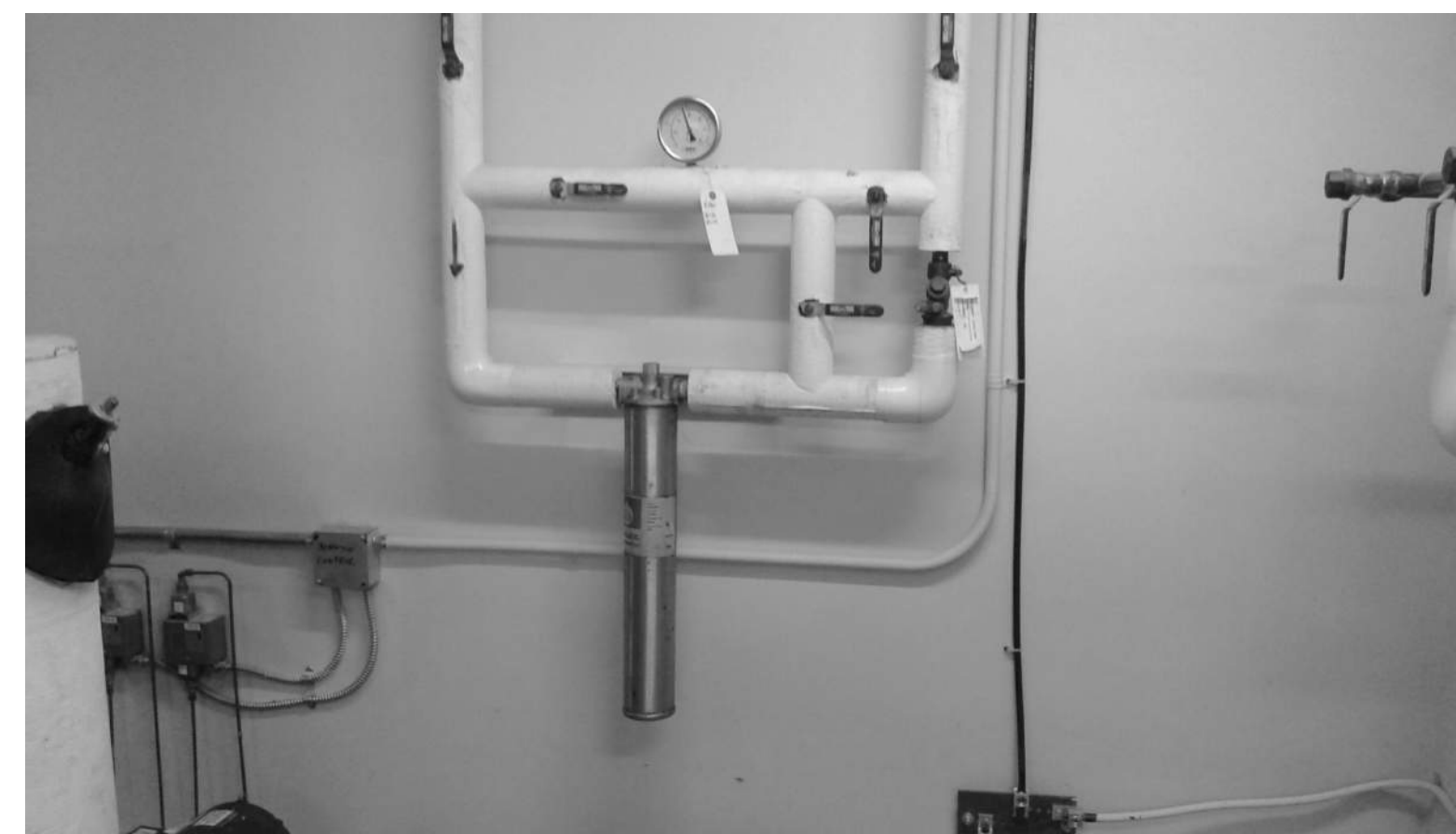
CHEMICAL FEED PIPING
