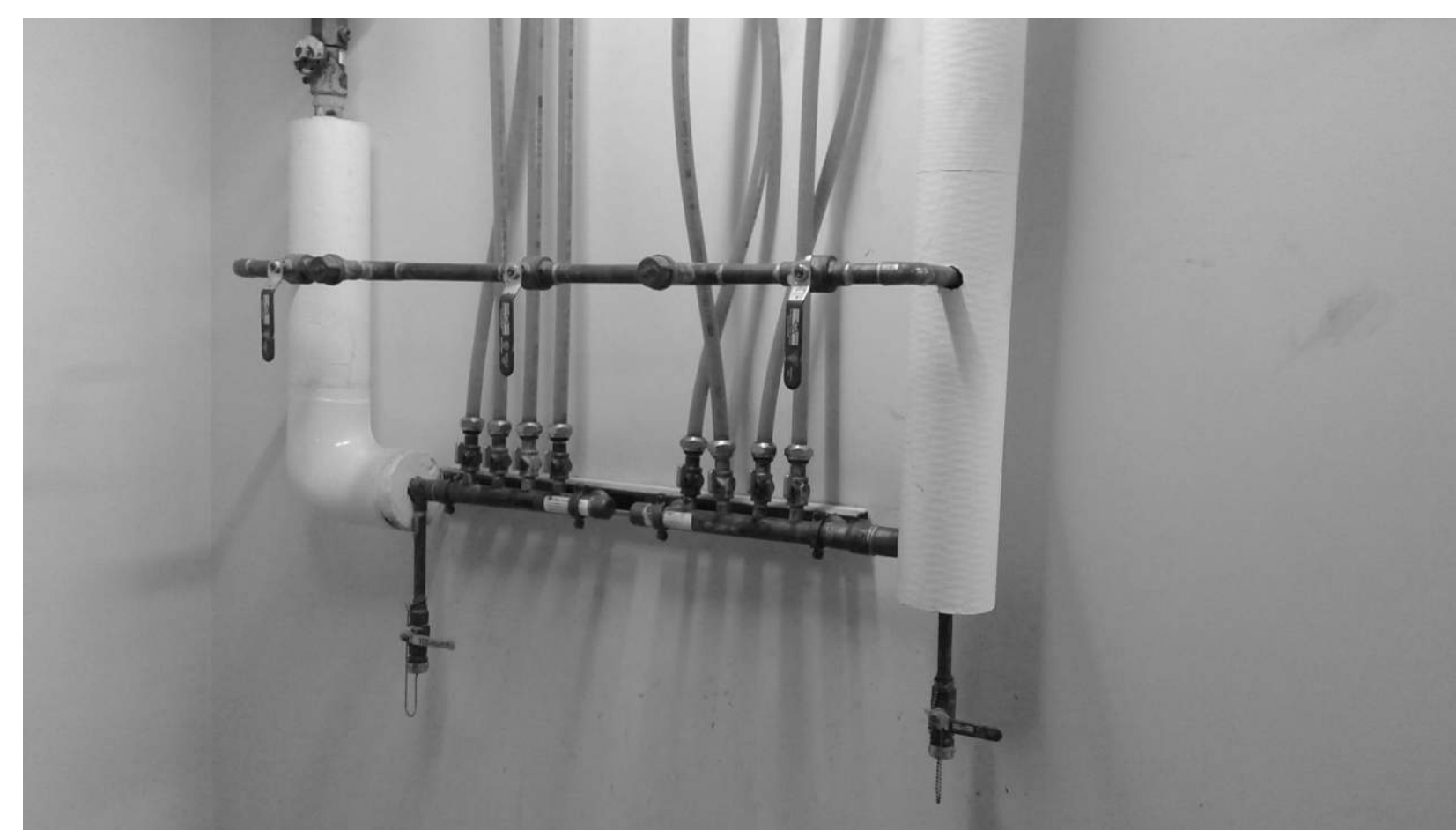
SNOW MELT MANIFOLD
