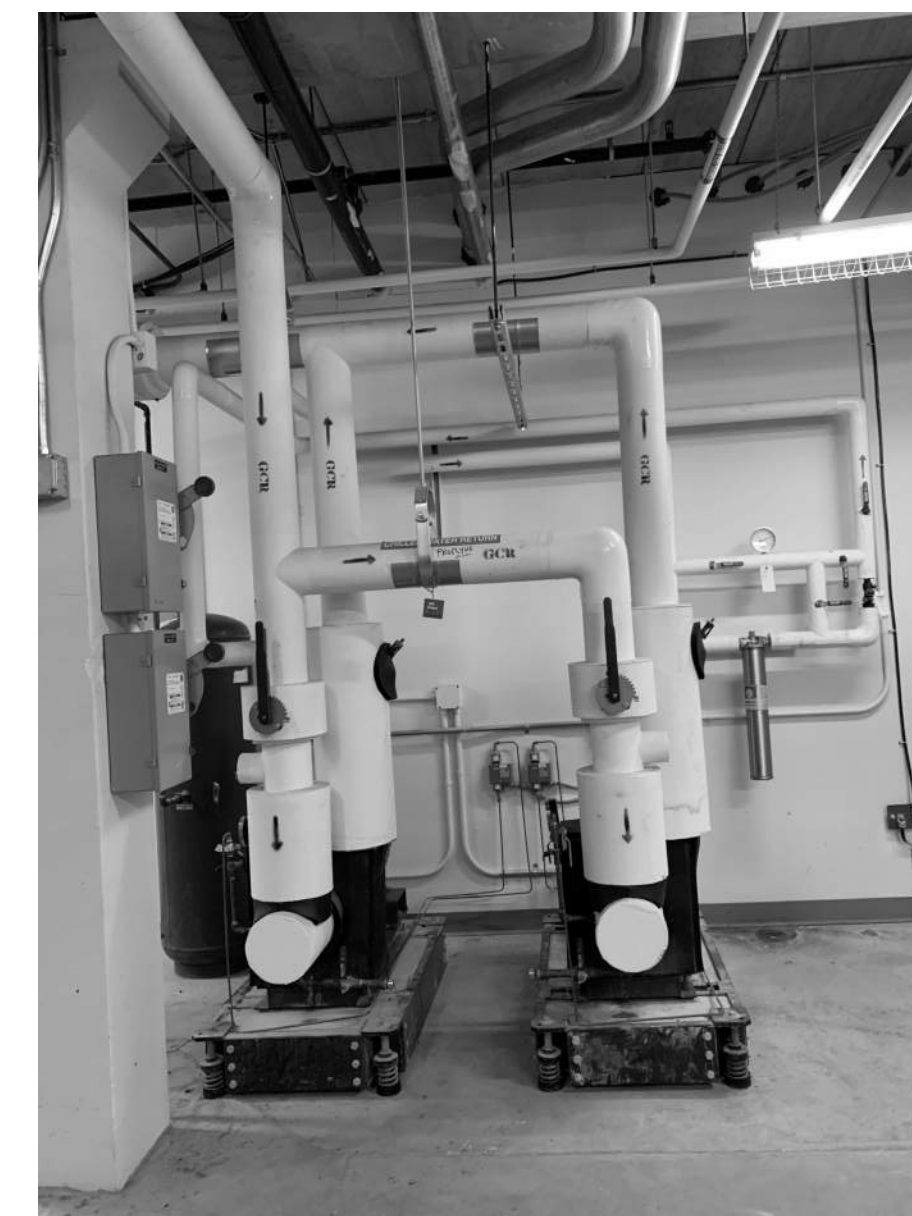
GLYCOL CHILLED WATER PIPING (LOOKING SOUTH)
