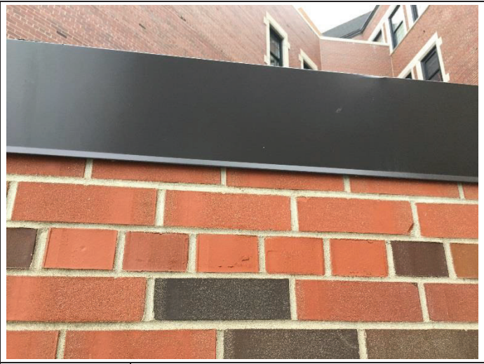
PHOTO 26 Black Flashing - Exterior <1mg/cm 2 lead
