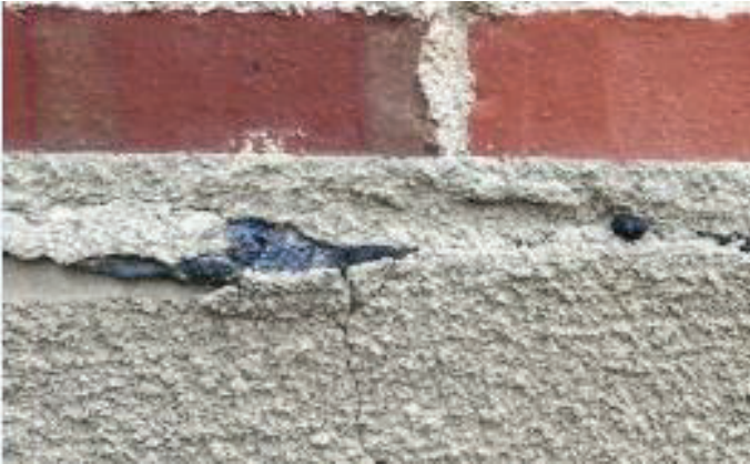
PHOTO 7 Black Tar Under EFIS – Mech. Room Entry
