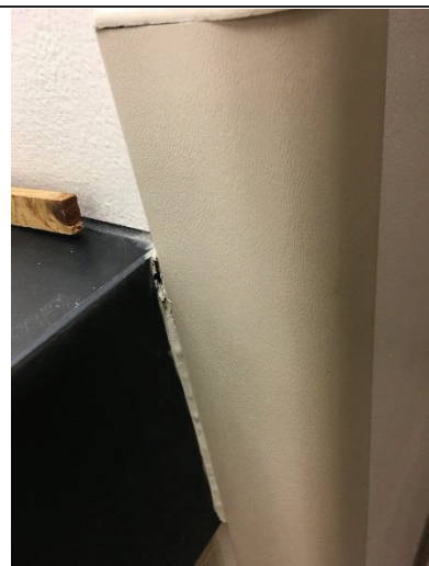
PHOTO 36 White Mastic – Lab Base Cabinets
