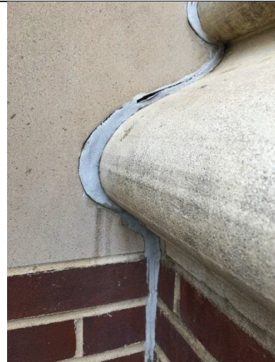
PHOTO 14 Gray Joint Caulk - Exterior
