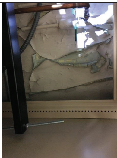
PHOTO 75 Peeling White Paint Under Sink <1mg/cm 2 lead
