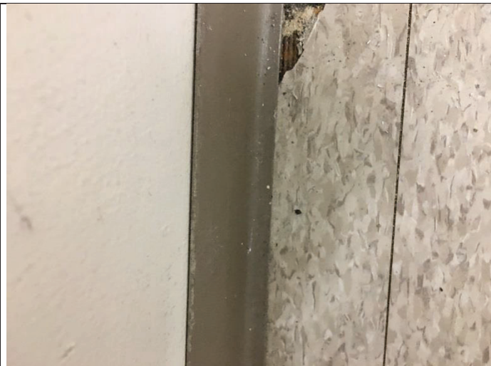
PHOTO 41 12" x 12" VFT Tan Blotchy/Mastic Black Mastic 4% Chrysotile
