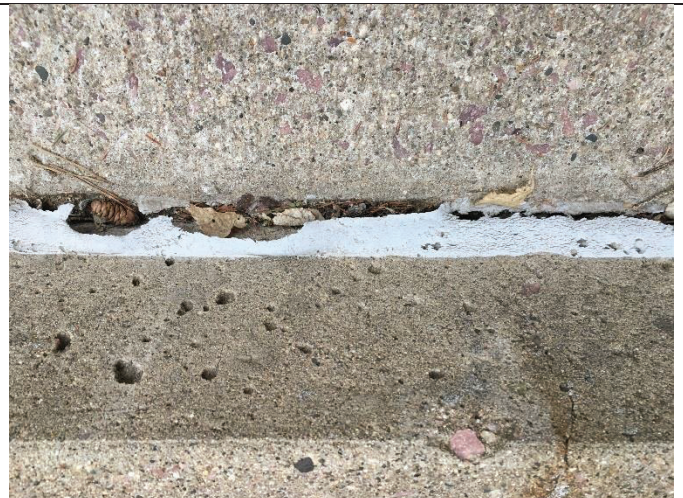
PHOTO 12 Gray Joint Caulk – Horizontal Concrete Pad
