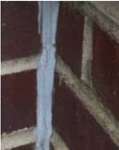
PHOTO 15 Gray Joint Caulk - Exterior
