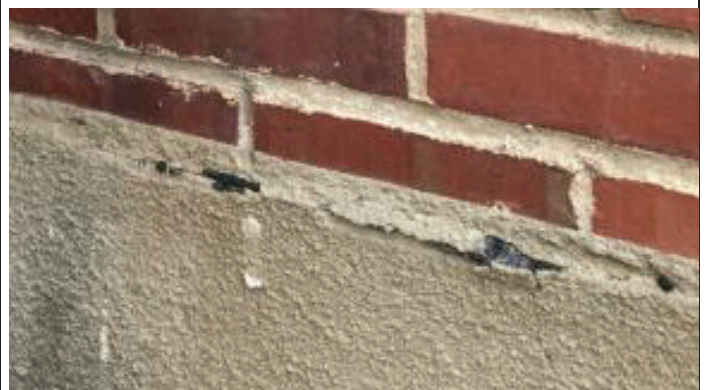
PHOTO 6 Black Tar Under EFIS – Mech. Room Entry
