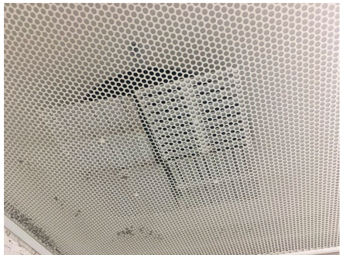
PHOTO 54 Diffuser Grate – Hallway by D-17 <1mg/cm 2 lead
