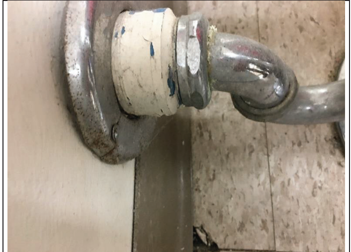
PHOTO 40 12" x 12" VFT Tan Blotchy/Mastic Black Mastic 4% Chrysotile
