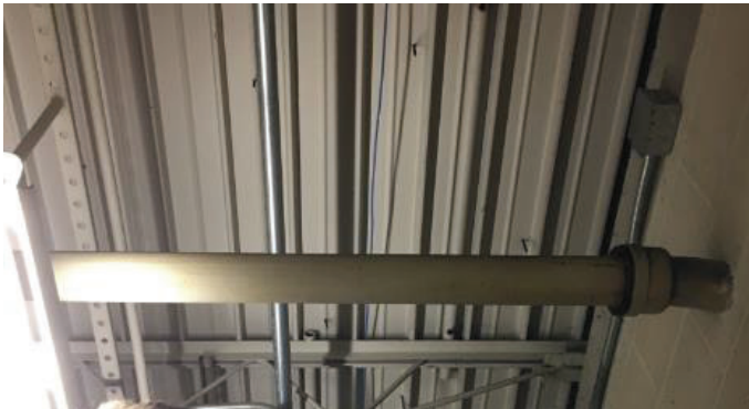
PHOTO 17 White Painted Pipe – Below Grade Mech. Room <1mg/cm 2 lead
