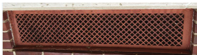
PHOTO 27 Red Ventilation Duct - Exterior <1mg/cm 2 lead
