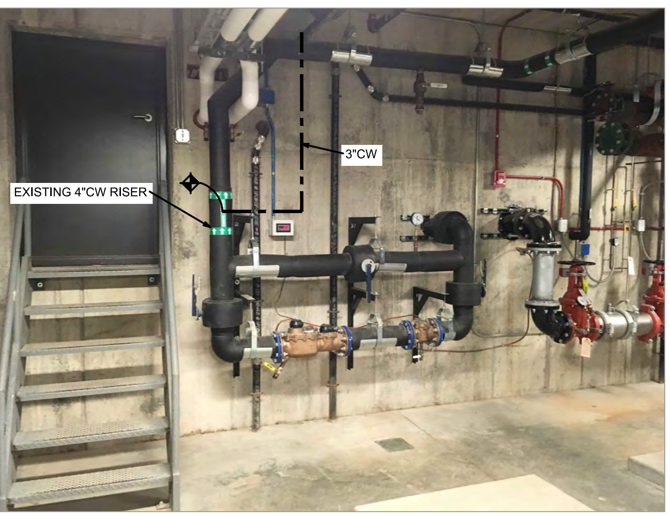
C6 EXISTING REHAB BUILDING WATER SUPPLY NTS
