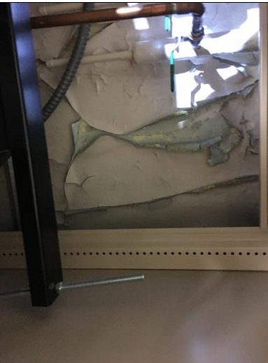
PHOTO 75 Peeling White Paint Under Sink <1mg/cm 2 lead
