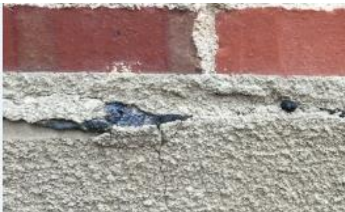
PHOTO 7 Black Tar Under EFIS – Mech. Room Entry
