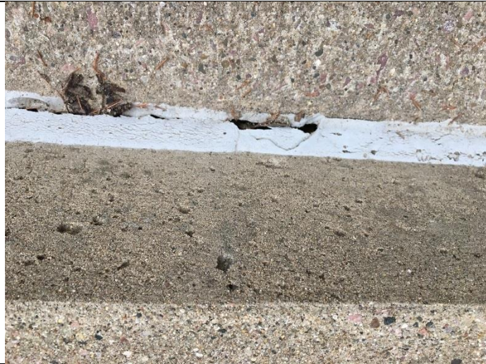
PHOTO 13 Gray Joint Caulk – Horizontal Concrete Pad
