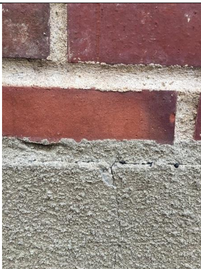
PHOTO 5 EFIS Surfacing – Mech. Room & Entry Area
