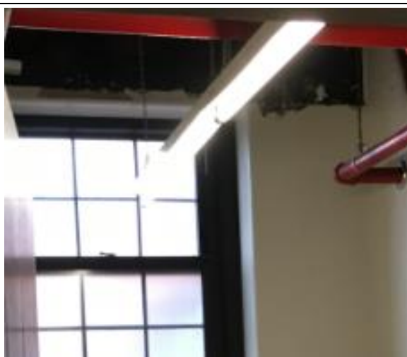
PHOTO 88 Black Concrete Wall Above Window – D-20 <1mg/cm 2 lead
