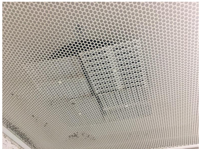
PHOTO 54 Diffuser Grate – Hallway by D-17 <1mg/cm 2 lead
