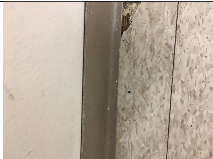
PHOTO 41 12" x 12" VFT Tan Blotchy/Mastic Black Mastic 4% Chrysotile
