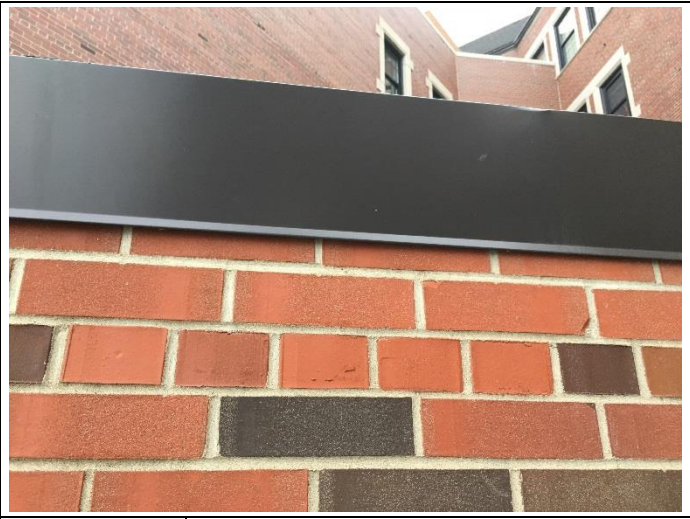
PHOTO 26 Black Flashing - Exterior <1mg/cm 2 lead
