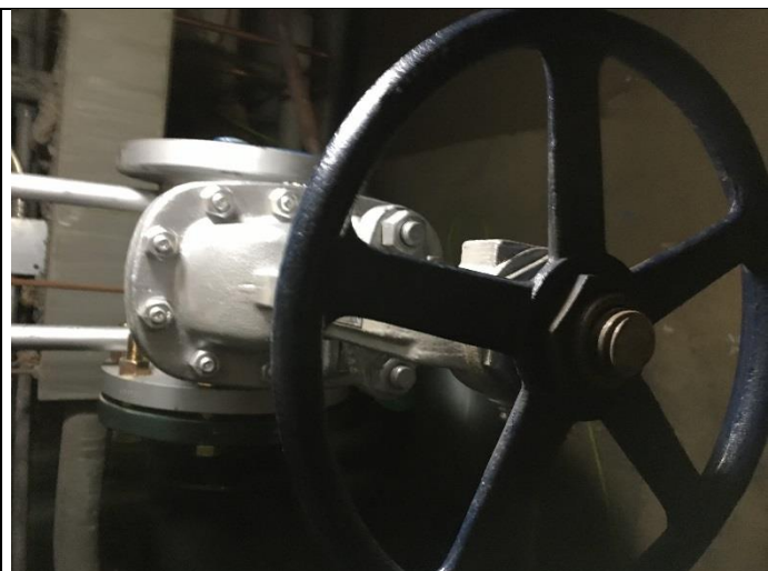
PHOTO 42 Silver Valve - Tunnel <1\text{ mg/cm}^2 lead
