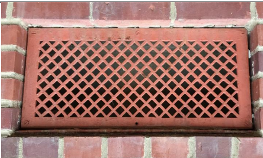
PHOTO 29 Red Decorative Grate on vertical wall - exterior 10.2 mg/cm 2 lead
