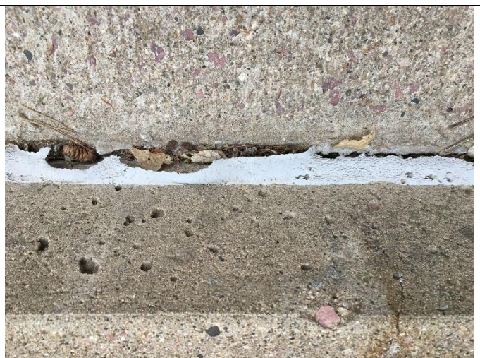
PHOTO 12 Gray Joint Caulk – Horizontal Concrete Pad
