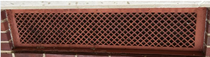
PHOTO 27 Red Ventilation Duct - Exterior <1mg/cm 2 lead
