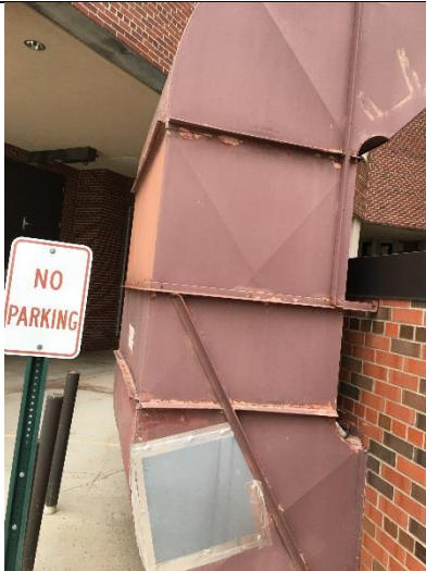
PHOTO 27 Red Ventilation Duct - Exterior <1mg/cm 2 lead
