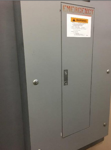
PHOTO 83 Breaker Box – D-20 <1mg/cm 2 lead
