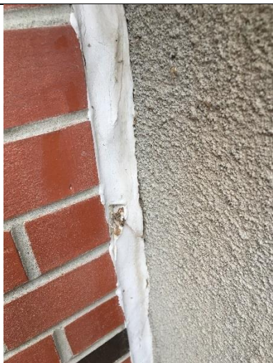
PHOTO 9 White Joint Caulk – Entry to Mech. Room
