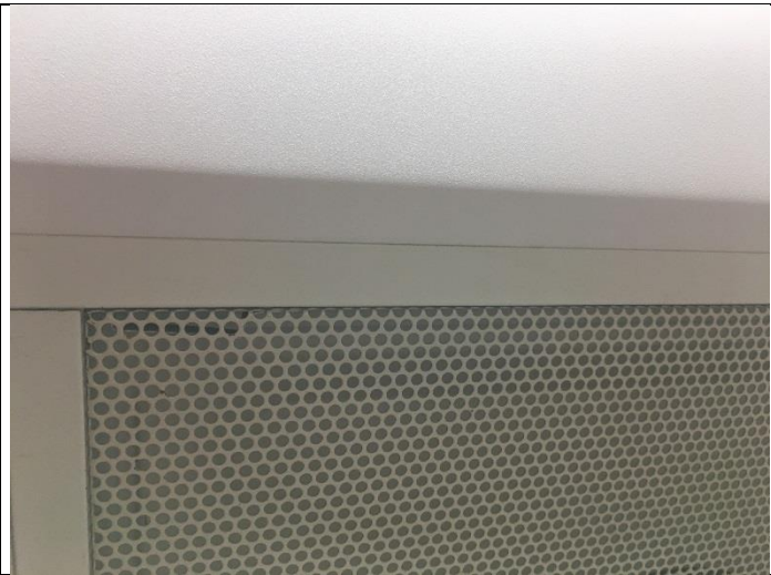
PHOTO 55 Ceiling Grid Hallway by D-17 <1mg/cm 2 lead
