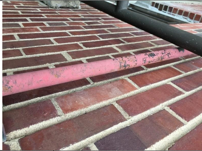
PHOTO 25 Red Pipe - Exterior <1mg/cm 2 lead
