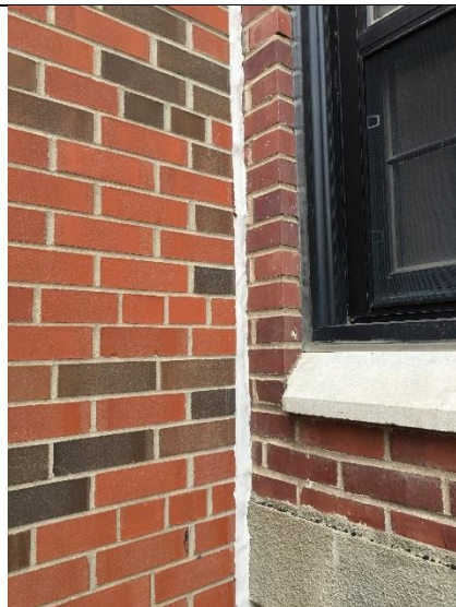
PHOTO 8 White Joint Caulk – Entry to Mech. Room
