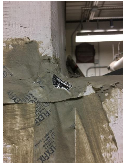
PHOTO 2 Gray Mastic – Duct in below grade mechanical room
