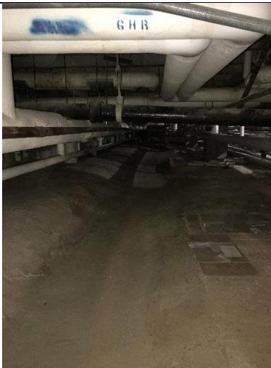
PHOTO 34 Black Pipe – Tunnel <1mg/cm 2 lead
