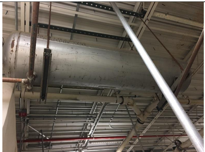
PHOTO 18 Silver Overhead Tank – Below Grade Mech. Room <1mg/cm 2 lead
