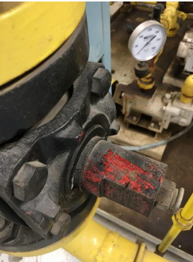
PHOTO 33 Building 2 Subgrade to Boiler Room 3-Black/Red under painted valves <0.5% Lead
