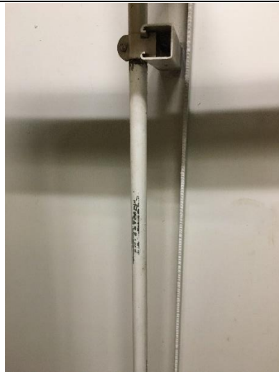
PHOTO 14 Building 2 Boiler Room 1" Gray Pipes <0.5% Lead
