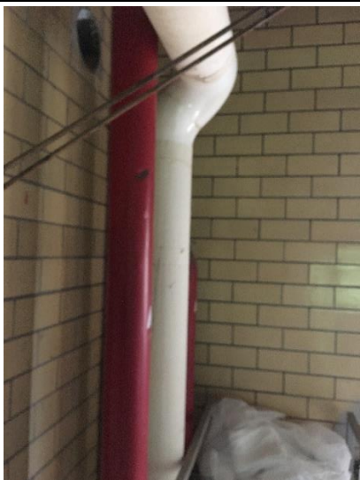
PHOTO 7 Red Jacketed TSI on Pipe Assumed ACM
