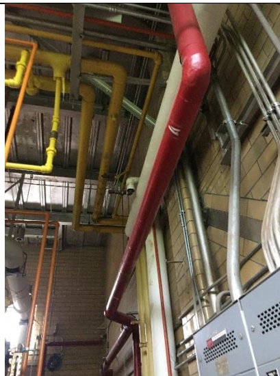
PHOTO 8 Red Jacketed TSI on Pipe Assumed ACM
