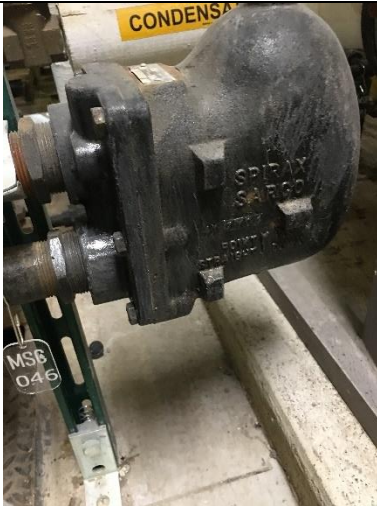
PHOTO 1 Building 1 – B024 Below Grade Mechanical Room <0.5% lead
