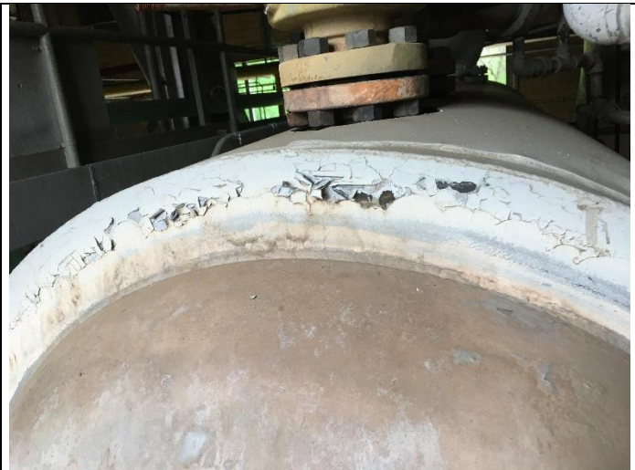
PHOTO 16 Building 2 Boiler Room Edge strip paint 1&2 >0.5% lead
