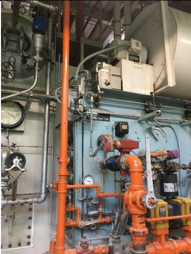
PHOTO 11 Building 2 Boiler Room Blue Paint on Boilers 1&2 >0.5% lead
