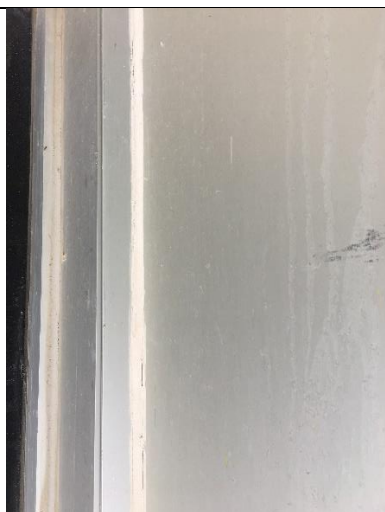
PHOTO 11 Gray Window Caulk – Exterior Non-ACM
