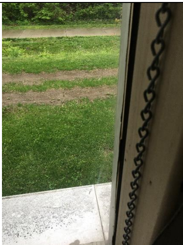
PHOTO 3 Caulk on interior side of windows Building 2 Boiler Room Non-ACM
