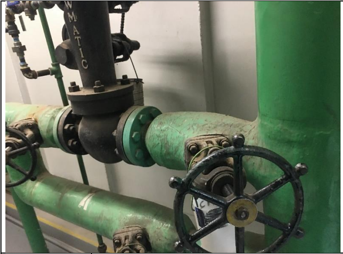
PHOTO 19 Green Jacketed TSI on Pipe Assumed ACM
