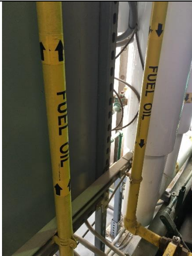
PHOTO 31 Building 2 Boiler 3-Yellow Fuel Line <0.5% lead
