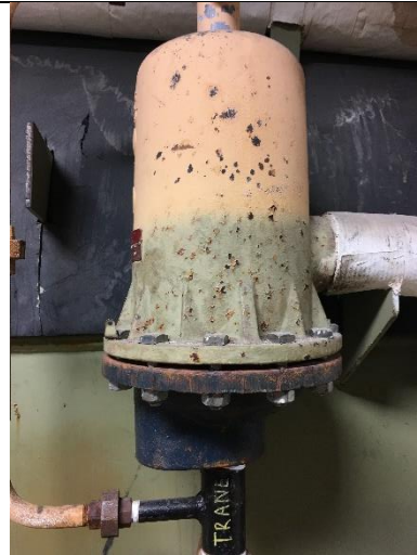
PHOTO 4 Building 1 Chiller Room Across from Mechanical Room B024 <0.5% lead
