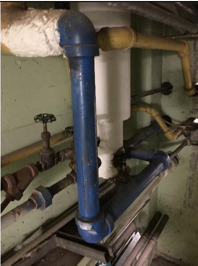
PHOTO 35 Building 2 Subgrade to Boiler Room 3-Blue painted <0.5% Lead
