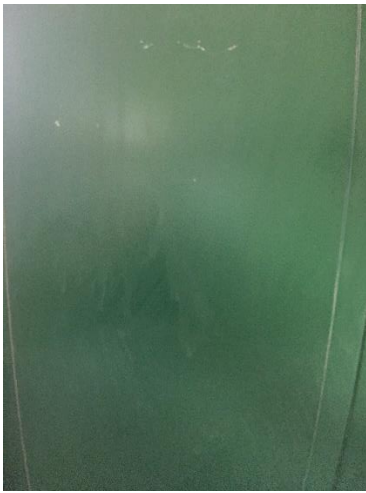
PHOTO 27 Building 2 – Green Painted Boiler 3 <0.5% lead
