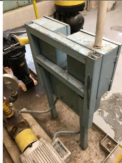
PHOTO 32 Building 2 Subgrade Below Boiler 3-Blue Control box/valves <0.5% lead
