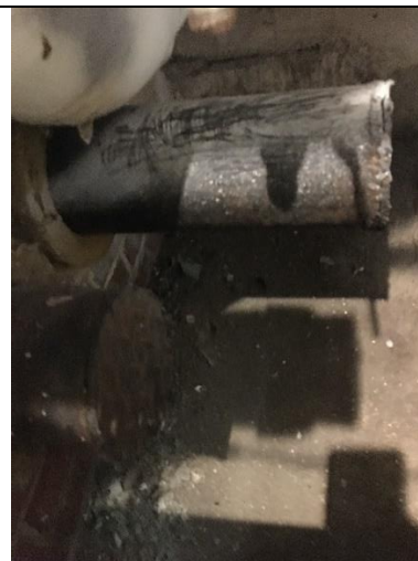
PHOTO 10 Debris on Floor under Glycol Pipes Non-ACM
