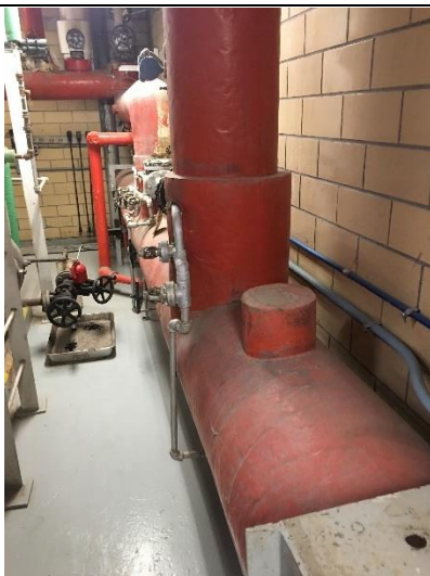
PHOTO 5 Red Jacketed TSI on Pipe Assumed ACM
