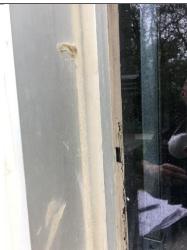
PHOTO 12 Brown Window Caulk – Exterior Non-ACM
