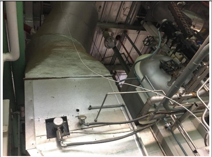
PHOTO 22 Silver Painted Flue Assumed ACM
