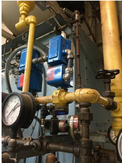
PHOTO 13 Building 2 Boiler Room - Yellow Pipes <0.5% Lead
