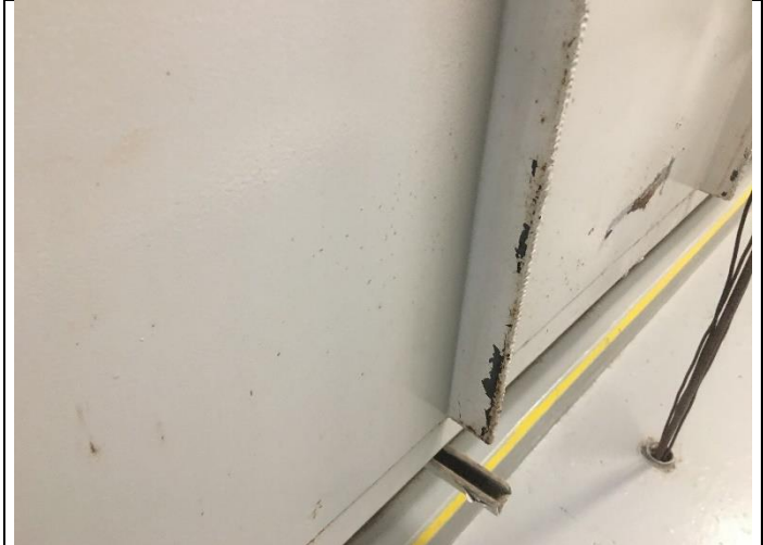
PHOTO 8 Building 2 Boiler Room – Gray Paint (Boiler 1) >0.5% Lead
