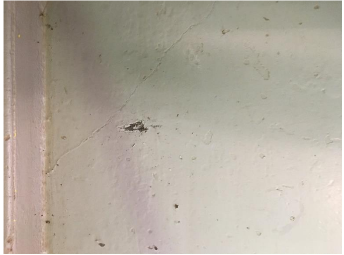
PHOTO 38 Building 2-Gray Painted Boiler Room Floor <0.5% Lead
