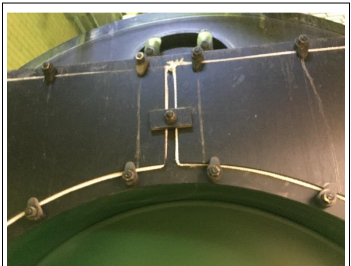
PHOTO 24 White Gasket on Boiler 3 Ends Non-ACM
