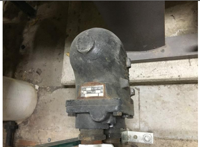
PHOTO 2 Building 1 – B024 Below Grade Mechanical Room <0.5% lead
