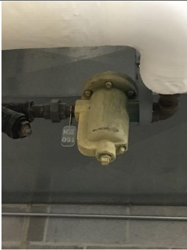
PHOTO 7 Building 1- Mechanical Room 716 <0.5% lead
