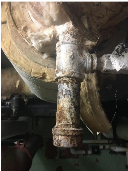
PHOTO 1 Residual TSI on Drip Leg Non-ACM
