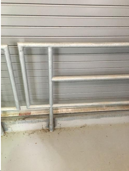
PHOTO 37 Handrail in front of OH Door <0.5% Lead
