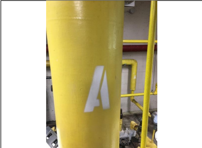
PHOTO 13 Yellow Jacketed TSI on Pipe Assumed ACM
