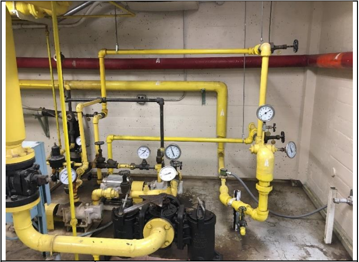
PHOTO 16 Yellow Jacketed TSI Fittings Assumed ACM
