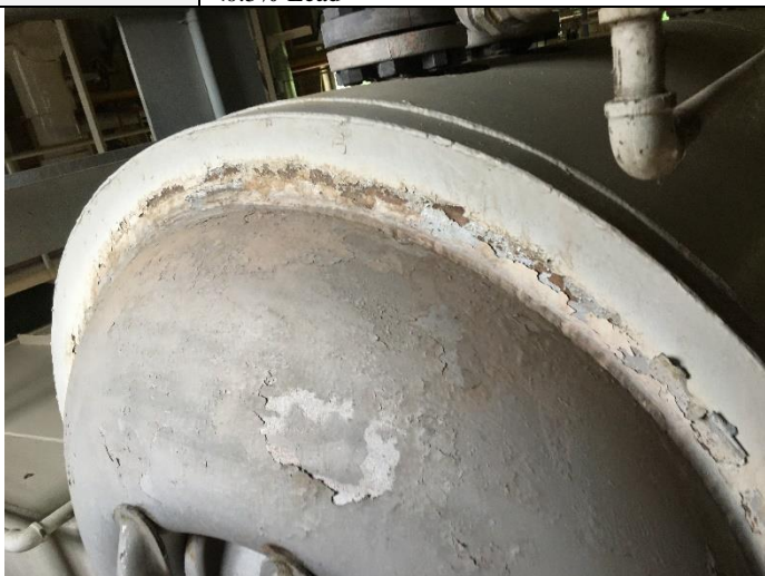
PHOTO 17 Building 2 Boiler Room – Boiler End Dome <0.5% Lead
