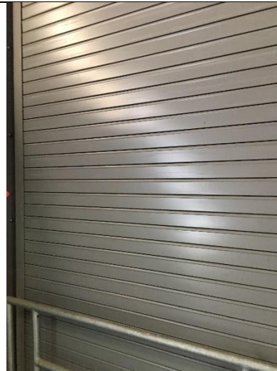
PHOTO 36 Building 2 Boiler 3-Gray OH Door/Frame <0.5% lead
