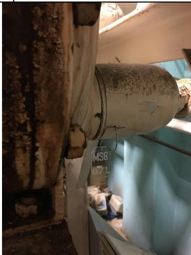
PHOTO 5 Building 1 Chiller Room Across from Mechanical Room B024 <0.5% lead
