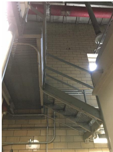
PHOTO 15 Building 2 Boiler Room Stairs/Platform <0.5% Lead
