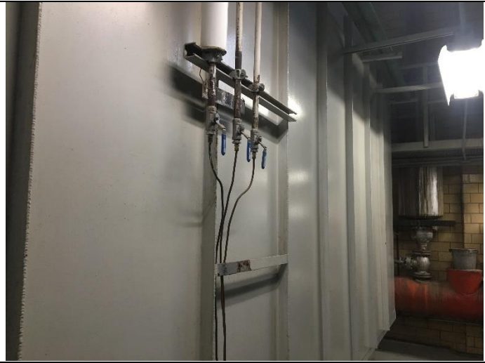
PHOTO 9 Building 2 Boiler Room – Gray Paint (Boiler 2) <0.5% Lead
