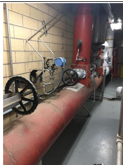
PHOTO 6 Red Jacketed TSI on Pipe Assumed ACM
