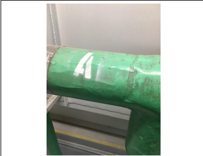
PHOTO 17 Green Jacketed TSI on Pipe Assumed ACM
