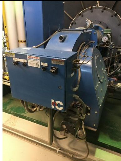
PHOTO 26 Building 2 – Boiler Room Boiler 3 Blue Painted Frame/Controls <0.5% Lead
