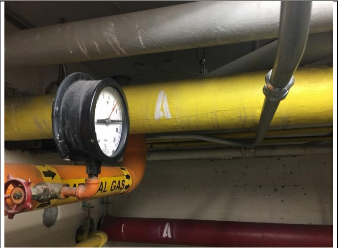
PHOTO 14 Yellow Jacketed TSI on Pipe Assumed ACM
