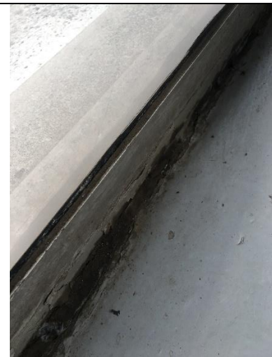
PHOTO 4 Caulk on interior side of windows Building 2 Boiler Room 6% Chrysotile
