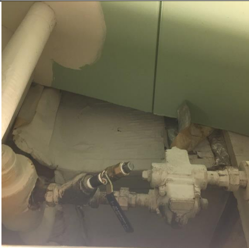
PHOTO 3 Building 1 B024 – Below Grade Mechanical Room <0.5% lead
