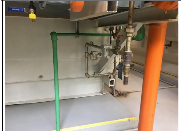
PHOTO 12 Building 2 Boiler Room Green Painted Pipes <0.5% Lead
