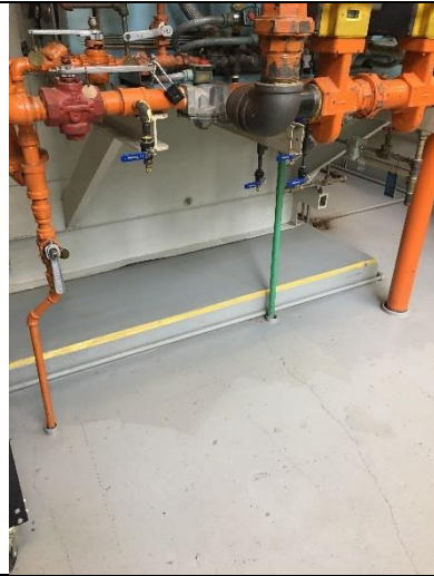
PHOTO 10 Building 2 Boiler Room Orange Painted Pipe >0.5% lead
