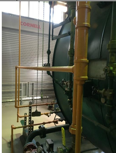
PHOTO 29 Building 2 Boiler Room 3 Orange/Yellow 1 1/2” Gas Lines <0.5% lead
