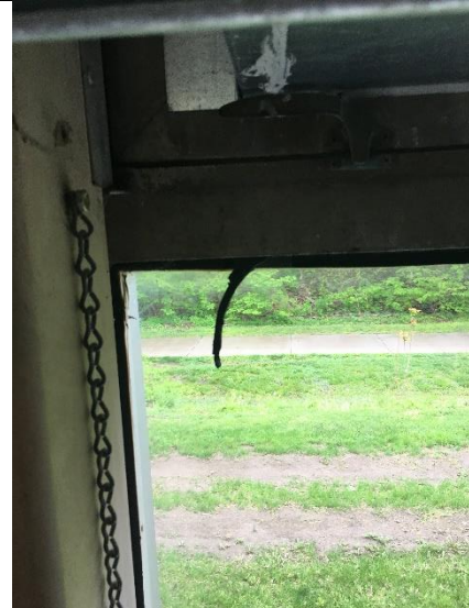
PHOTO 2 Caulk on interior side of windows Building 2 Boiler Room 6% Chrysotile
