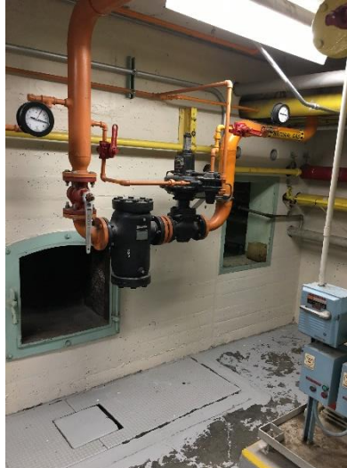
PHOTO 34 Building 2 Subgrade to Boiler Room 3-Black painted valves >0.5% Lead
