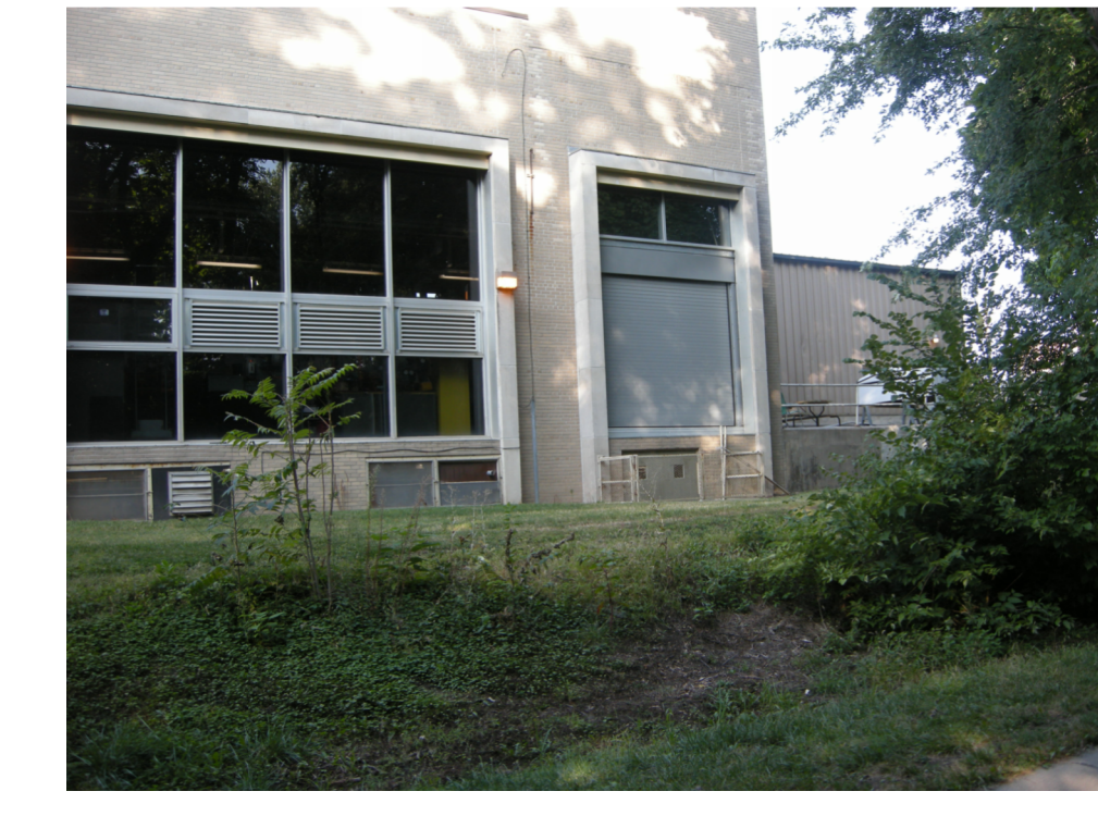
A8 EXISTING CONDITION ALONG EAST WALL N.T.S.
