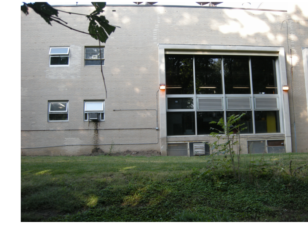
A7 EXISTING CONDITION ALONG EAST WALL N.T.S.
