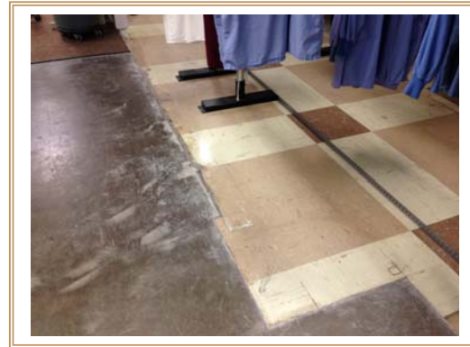
View of significantly damaged, asbestos-containing , cut 9"x9" floor tiles/mastic. Building 5, ground level, room E06.
