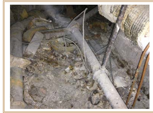
View of significantly damaged asbestos-containing pipe insulation and mudded fittings. Building 1, basement, underfloor crawlspace areas.
