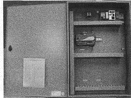
FEC/IOM Standard Control Panel Assembly Mounted in a 24 in. x 36 in. Enclosure
