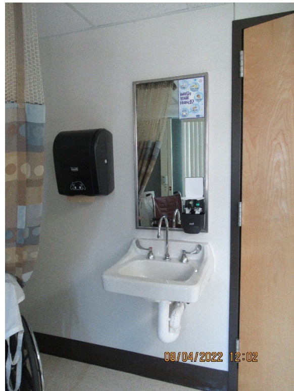
Figure 8: Bld. 48 Room 106C sink and plumbing
