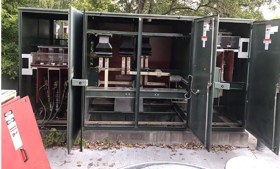
Figure 3. – Existing Exterior 25 KV Switchgear
