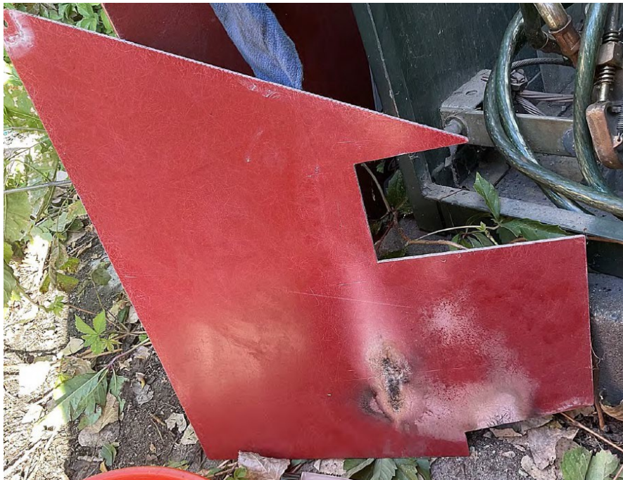
Figure 4. – Existing Exterior 25 KV Switchgear Barrier To Reinstall If Repair In Place Option Is Selected
