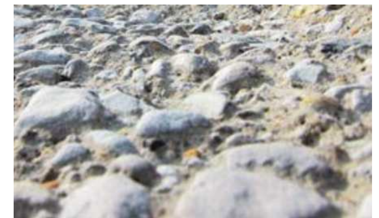
FIGURE A CSP 10 SURFACE CHARACTERISTICS - SURFACE PREPARED USING HANDHELD CONCRETE BREAKER FOLLOWED BY ABRASIVE BLASTING
