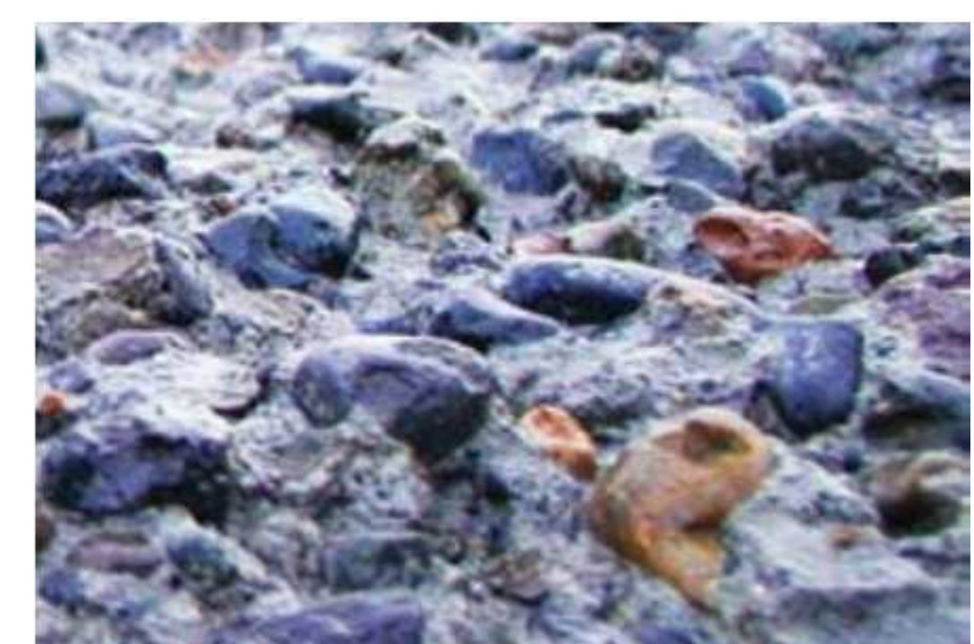
FIGURE B CSP 10 SURFACE CHARACTERISTICS - SURFACE PREPARED USING HIGH-PRESSURE WATER JETTING
