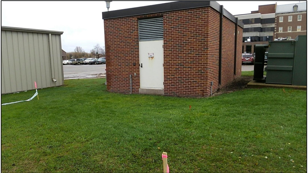
Photograph 1. Existing Site Facing Southeast
