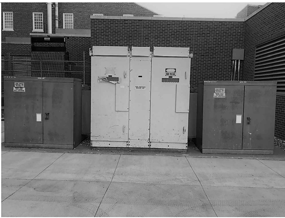
5 BUILDING 46 - TRANSFER SWITCH FEEDER 1 AND 2 ED1.02
